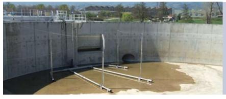
In larger tanks or for special applications, Grundfos RainJet systems can be designed with several outlets fed by a single pump.
